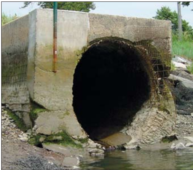
CSO outfall at Back Cove, Portland.
