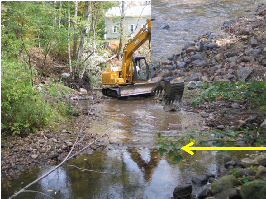
Temporary dam removed and feathering of stream bed
