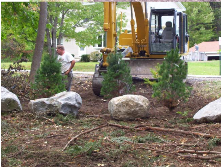
Access road also stabilized with brush, winter rye and hay.
