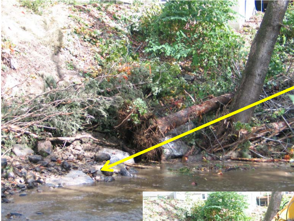
Rock vein with root wads packed around and behind.
