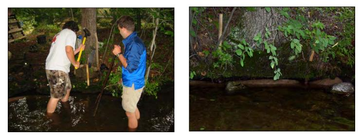
To prevent the undercutting from getting worse, "coconut roll" was installed in the eroded area. It is a mesh tube secured in place using wooden stakes. The tube will expand to fill the eroded area and keep the water from causing more damage.
