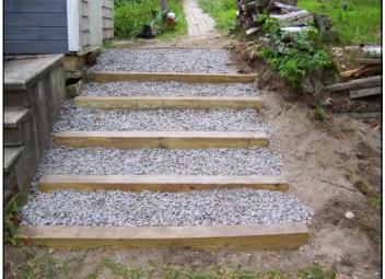
The retaining wall had collapsed most likely due to runoff from the brick path and rotting the wood. Five infiltration steps were installed to both slow down the runoff and prevent the exposed soil from washing into the water.
