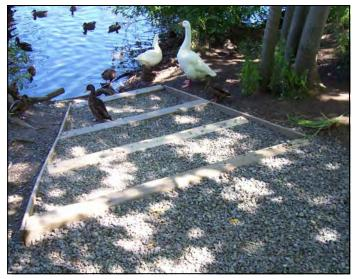
The infiltration steps installed at Riverbank Park by the 2007 PRYCC crew had been almost completely emptied of crushed rock. The crew re-filled the three sets of steps and added a new step to this set to reduce the steepness and allow more water to infiltrate. Westbrook Public Works was very cooperative and provided the necessary materials.
