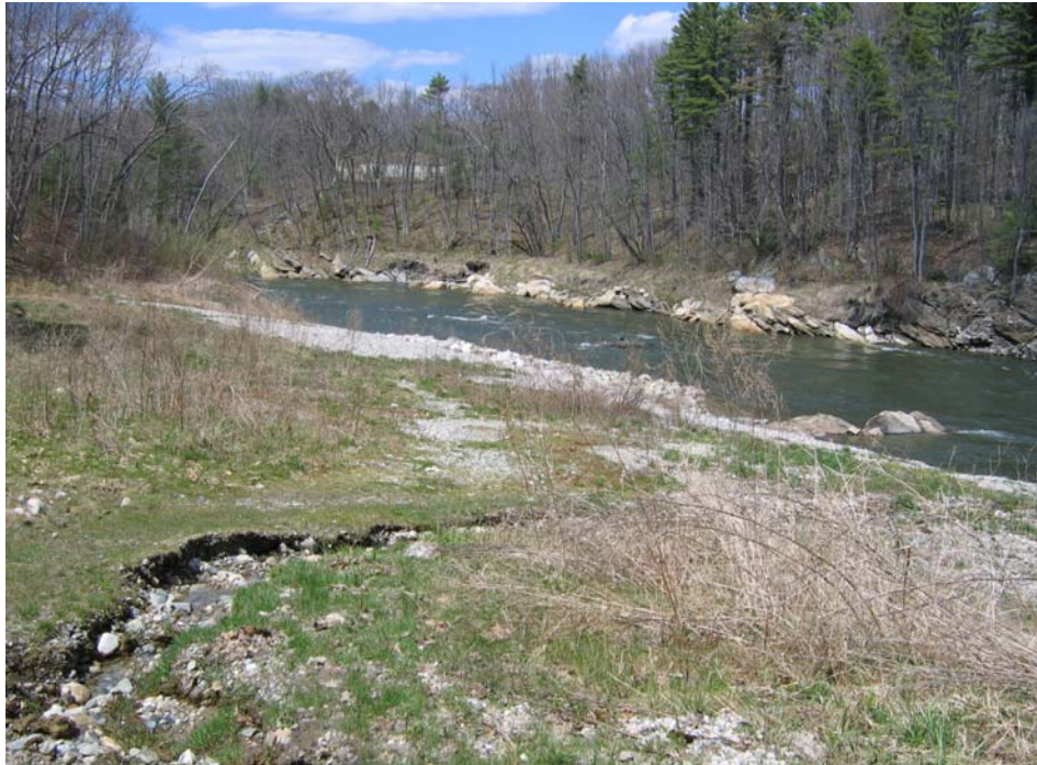
April 2005. Original stormwater runoff channel pre project implementation.
