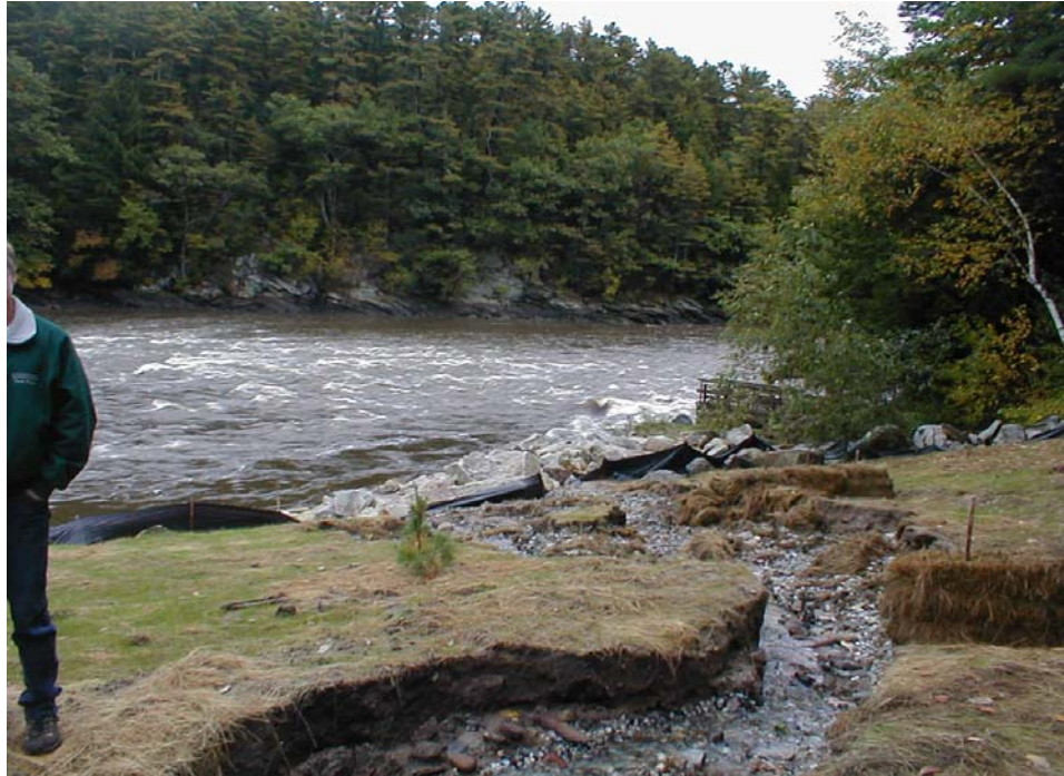
Fall 2005. Smelt Hill swale, lower run, after over 10 inches of rain falls in the area in one week.
