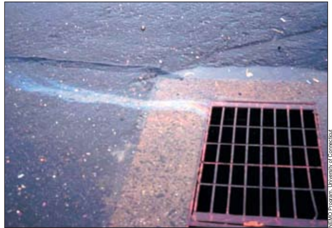
Impervious surfaces channel pollutants such as gasoline and oil into stormwater systems, which discharge into the rivers and streams flowing into Casco Bay.
