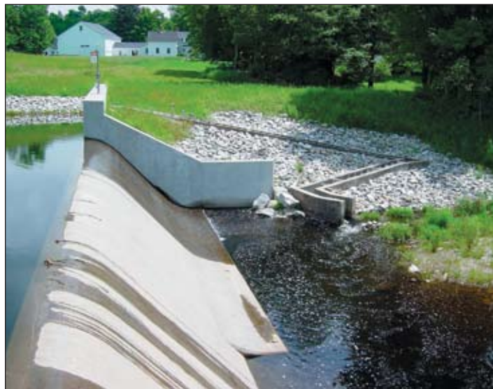
Crest of Highland Lake Dam and fishway with sediment bar obstructing attraction flow at fishway entrance. These improvements will help to restore runs of river herring and American eel.
