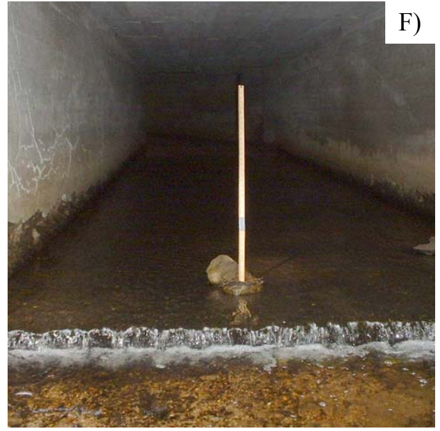
Site 1 photographs: A) scoured tree roots downstream of the Route 302 bridge/culvert; B) a woody debris dam and pool; C) a representative photograph of substrate in a run; D) trash on the streambank; E) alewives; and F) water level in the culvert (approx. 1 inch) (photo F taken on 7/14/03).
