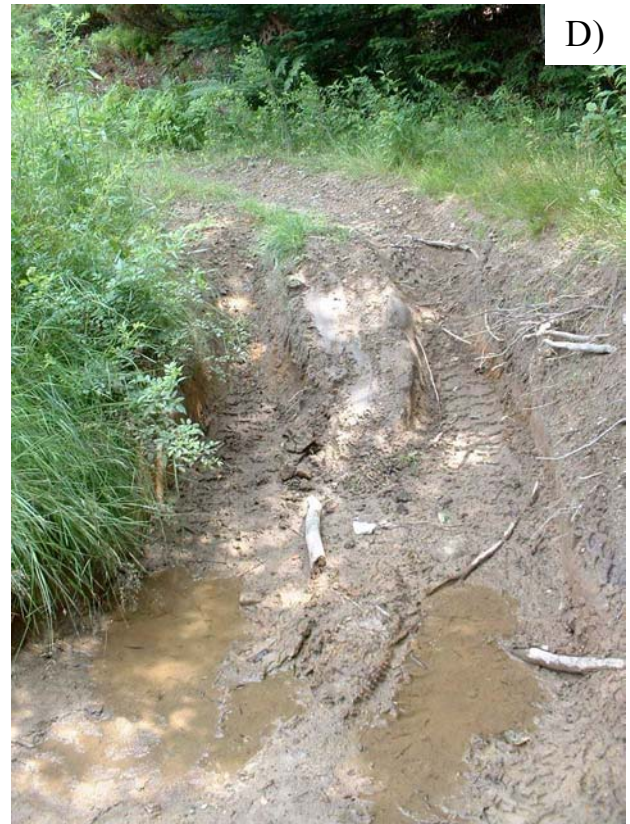
Site 4-B* photographs: A-B) signs of aggradation (that is, sediment accumulation or bar formation) in the middle of Mill Brook's channel and C-D) local ATV trail impacts. *These photos were taken on July 25, 2003, on a reconnaissance walk of this area.
