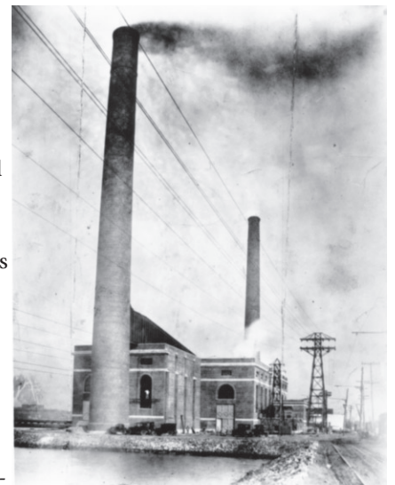
CMP STATION: Environmental regulations have reduced the amount of pollution released by industries and power plants like this one near the South Portland waterfront. But the legacies of the unregulated years may remain hidden in the soil, traveling in groundwater toward the harbor. (courtesy: Maine Historical Society)
