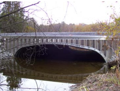
An open-bottom culvert is designed to restore water flow and fish passage in Thayer Brook in Gray, Maine.
