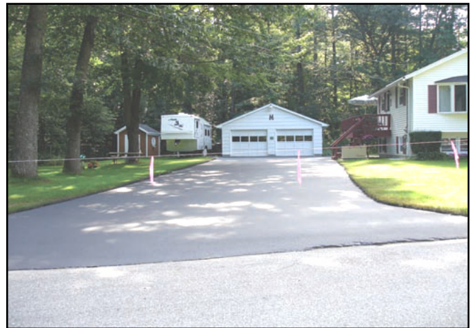
Recently seal-coated driveway in the Pleasant River Watershed; Stormwater picks up harmful polyaromatic hydrocarbons (PAHs) from seal-coating washing them into nearby streams and waterbodies.
