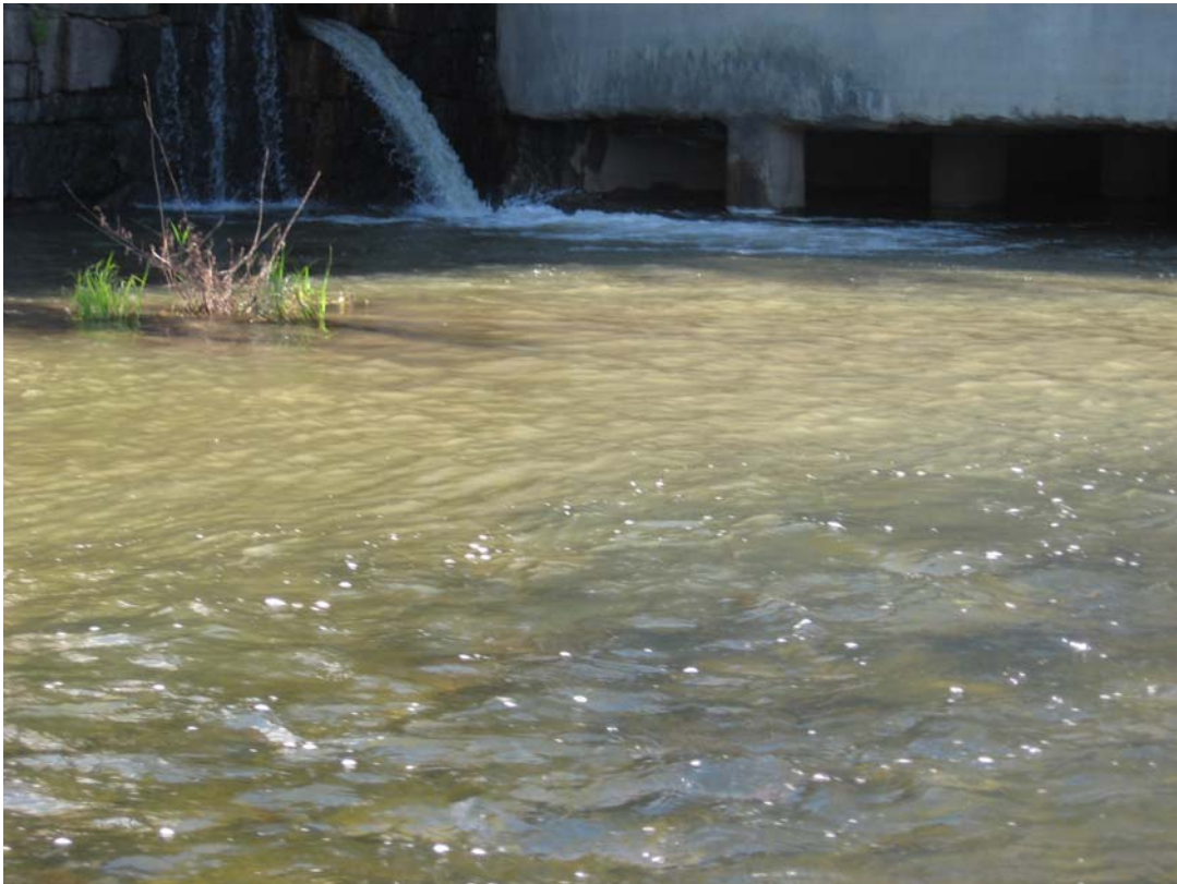
Plate 4. Discharge from the SAPPI facility immediately below the Cumberland Mills Dam observed on August 18, 2006. Note the turbidity plume resulting from suspended solids in the discharge.
