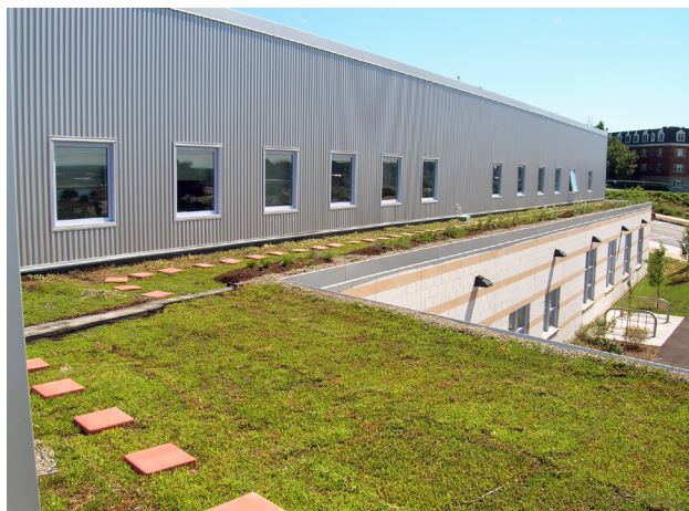
Green roof at the East End School in Portland.
