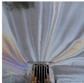
Oil entering a storm drain.
