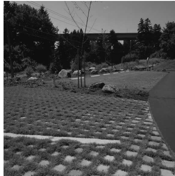
Concrete Grid Paver, Parking 2001 install 900 sq ft
